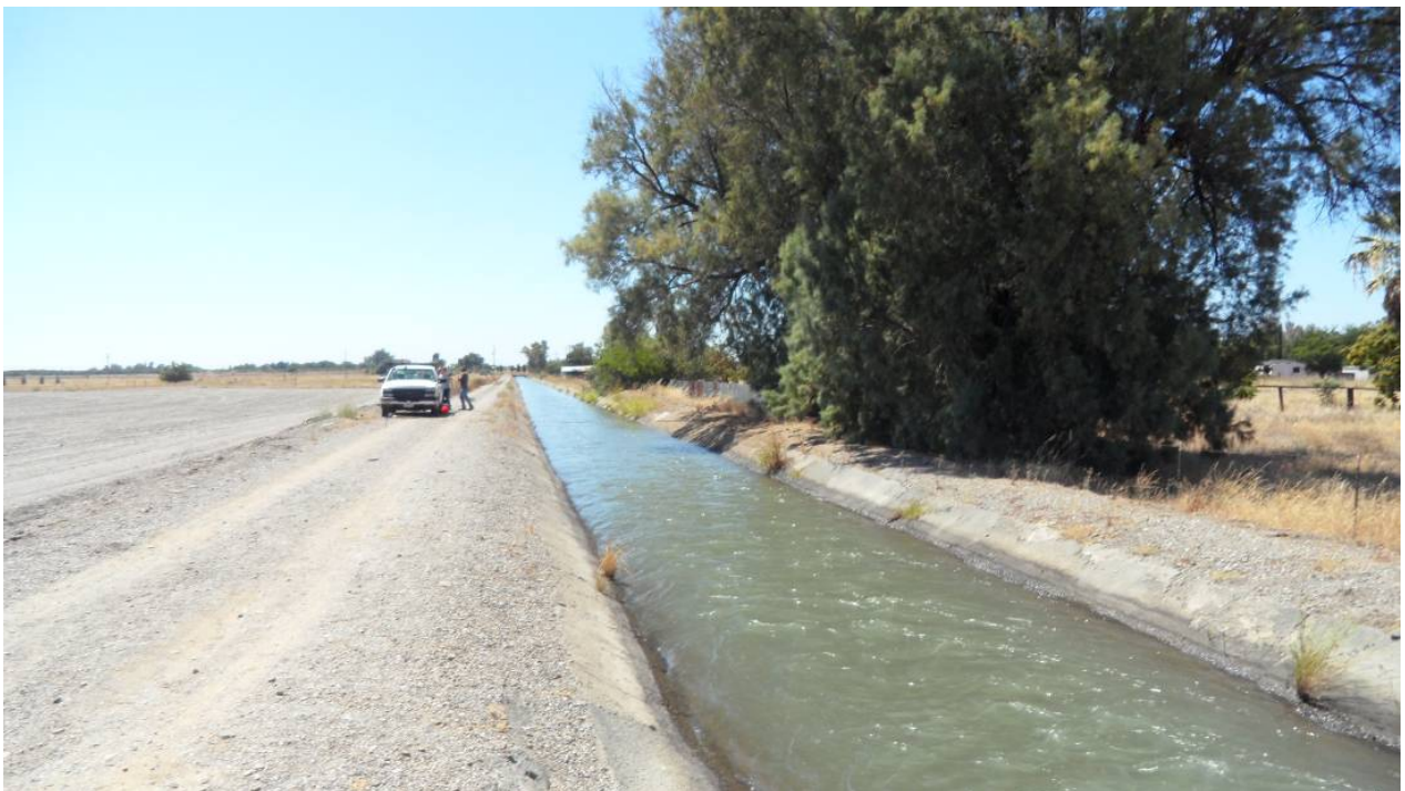
Figure 70. Good Installation Site: Long Straight Unobstructed Flow
